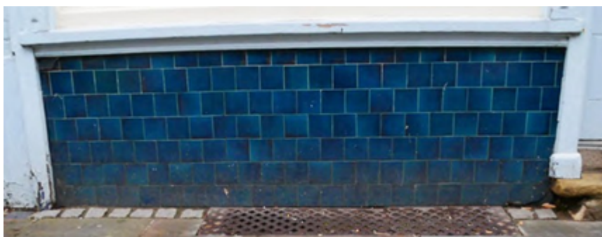
Figure 30 - Glazed blue tiles appropriate to this stallriser.
