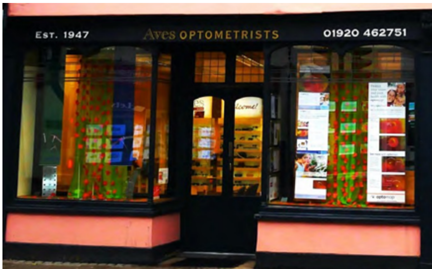
Figure 36- Appropriately scaled lettering to height of fascia.
